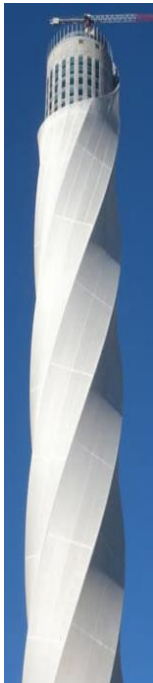
Fig.4-3: (left) Test tower [Jahn/Sobek] transverse vibration-avoiding GF fabric cover of the Thyssen-Krupp test tower for high-speed elevators Rottweil, 245m. (right) Mosque Masjid an Nabawi, Medina, sun protection 'umbrellas', Medina SA, 2010 [ILEK in cooperation with SL-Rasch]
