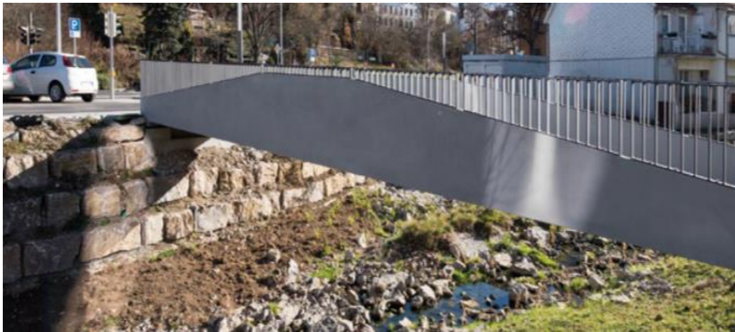
Fig.4-15: (up) a solidian GRID Q95-CCE-38 fiber grid (mat) [christian.kulas@solidian.com, www.solidian.com ] Thanks Christian (down) First, purely CF-reinforced concrete bridge in the world. Albstadt-Ebingen. 2015. According to (Construction) Mayor of Albstadt, Udo Hollauer, "The bridge pays off, and is sustainable"
