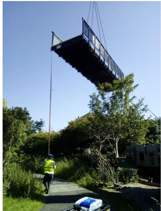
Fig.4-5: CFRP truss work production using a special strand placement (winding) technique and the fabricated bridge [BaltiCo GmbH, July 2020]. Thanks Dirk 25 m bicycle and pedestrian bridge made of CFRP in Sassnitz was installed, which was easier than usual due to the weight of just 1.4 tons of a single segment and took place within a single day. BaliCo Portfolio: Lattice masts, functionalized modular cabin plate elements, bridges, girders, lattice masts, telescopic towers, rotor blades.
