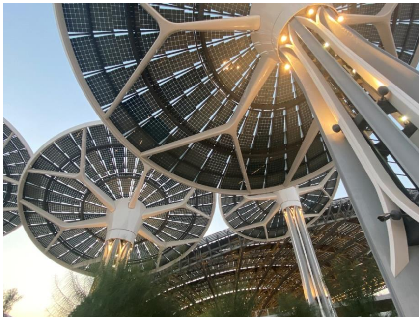
Fig.4.4-2 E-Trees Sustainability Pavilion: Light and stiff CFRP 'steering wheels' keep the load manageable for the mechanical rotation system that allows the E-trees to track the sun as the days progress to ensure that the up to 14 t of PV panels are always ideally positioned to maximize their efficiency.
