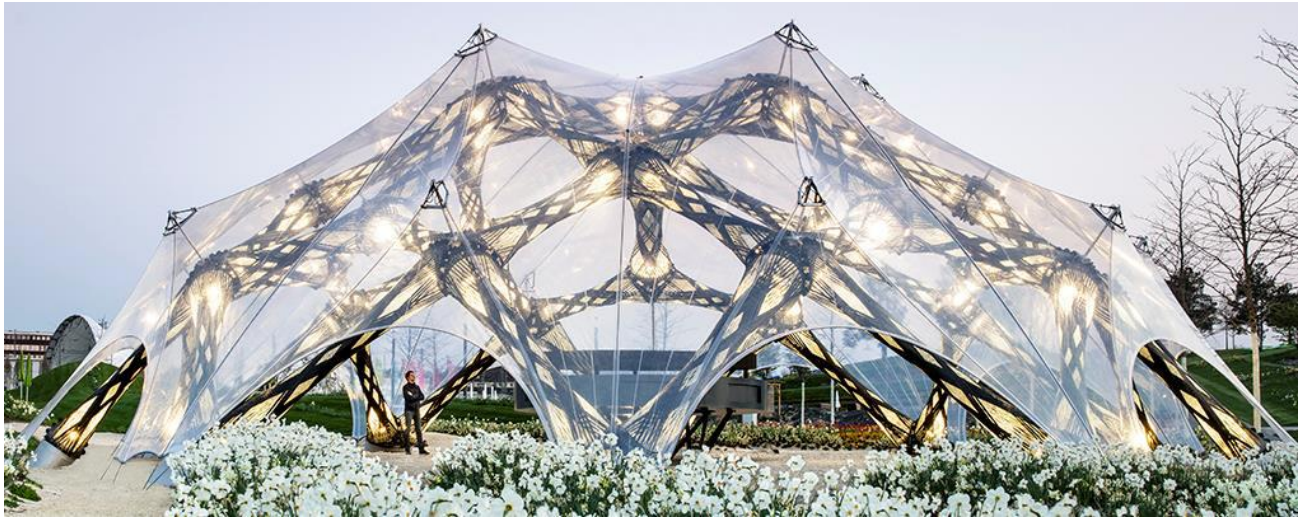
Fig.4-4: Special automated fabrication process with endless fiber strands ‘wound’ over the fixed 'truss' nodes as strand turning points. Lightweight 'fiber pavilion' made of 60 CFRP/GRP components, BUGA Heilbronn 2020. Art structure meets load-carrying structure [Knippers, Koslowski, ITKE Stuttgart; Menges, CD].
