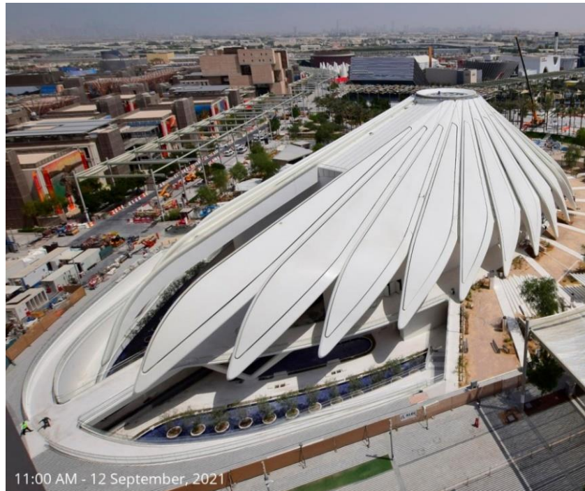
Fig.4.4-1 UAE Pavilion: FRP wings (built from a hybrid carbon and glass fibre build-up) and the claddings (built in glass fibre) resulted in an impressive 40% mass saving. The reduced mass was also beneficial during installation and allowed the entire wings to be hoisted in one piece. The wings were produced at PCT facilities to a maximum transportable size. Most wings were transported to the site already assembled – the larger ones arrived in two halves which were bolted together on-site and finished with a seamless joint. The repetitive nature of the FRP panels was critical for the effective use of tooling and cost-effective serial production of the wings and claddings. Furthermore, lamination schedule with curing procedure were optimized for each wing and for each zone to meet the structural requirements with a cost-effective approach
