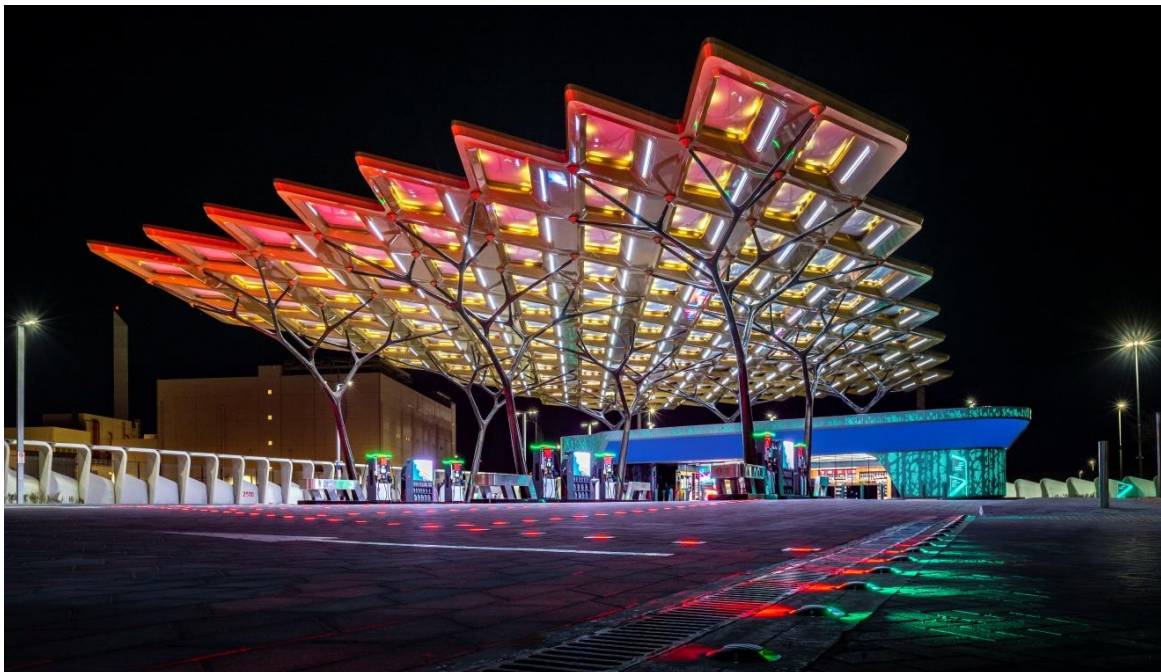
Fig.4.4-3 ENOC Petrol Station : CFRP was used to construct the entire structure of a service station canopy (roof) . It consists of 133 diamond shaped CFRP frames housing ETFE inflated cushions and photovoltaic panels. The entire structure is supported by an exoskeleton consisting of 9 slender molded CFRP Ghaf trees ( the tubes are built using filament winding with molded nodes manufactured from the same carbonfibre fabric).
