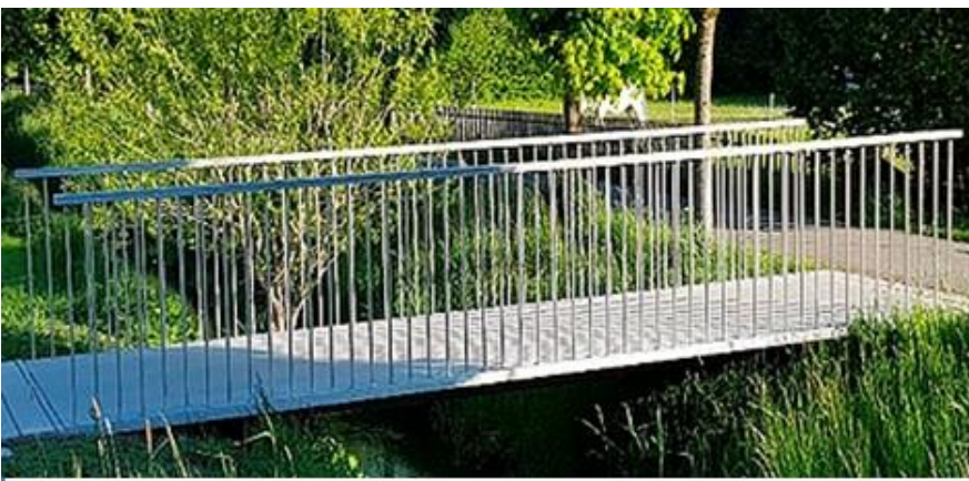
Fig.4-13: Hybrid bridge in Turbenthal made of pretensioned CPC slabs and CFRP beam supports. CPC-plate size: 2-7 cm thick, length 3.5 – 17 m [ZHAW, with J. Kurath]. Thanks Sepp
