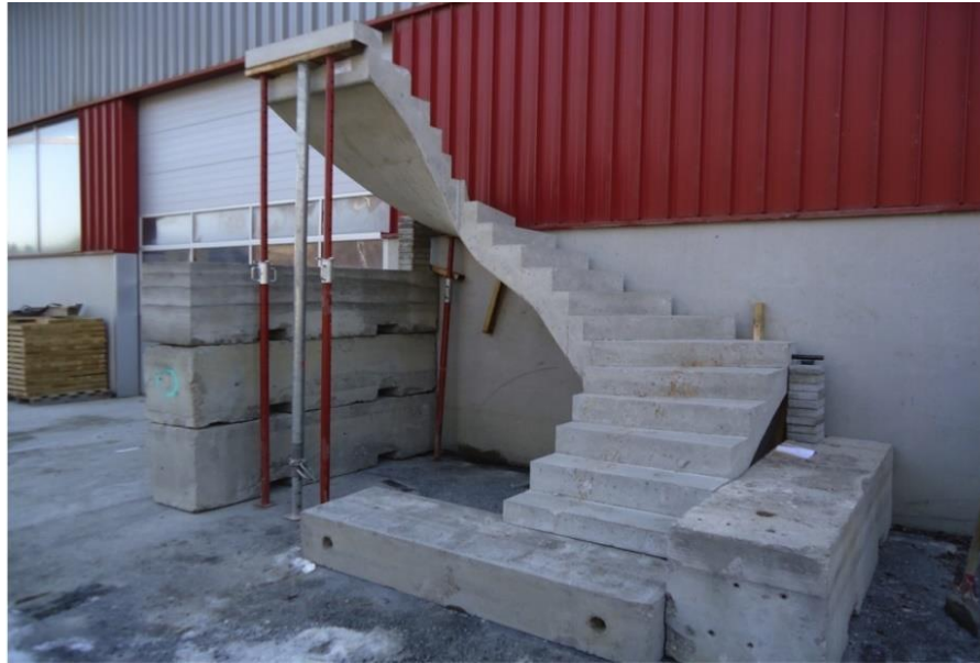
Fig.4-20: Staircase-Reinforcement with long steel fibers. [Faserbeton im Bauwesen, Springer, Bernhard Wietek. Thanks Bernhard]. What about long C-fibers?
