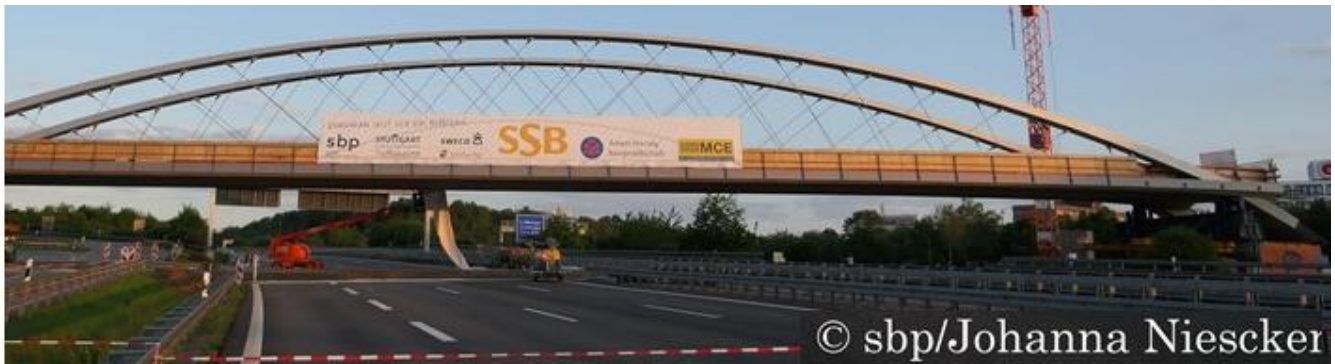
Fig.4-6: The Stuttgart Stadtbahn bridge, installed over the A8 motorway on May 3 in Germany, is the world's first network arch railway bridge (127 m) that hangs entirely on tension elements made of carbon fiber-reinforced plastic (CFRP). The 72 hangers are produced by Carbo-Link AG (Fehrltorf, Switzerland) supported by EMPA (Urs Meier), with Teijin carbon fibers (Wuppertal, Germany), Tenax. The bridge meets installation, mass and sustainability goal
