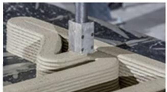
Project Milestone, City of Eindhoven [Freek Bos, Uni Eindhoven]
