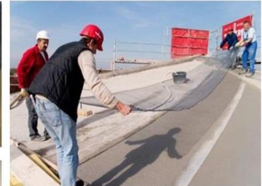
placing of a CF textile reinforcement mat
