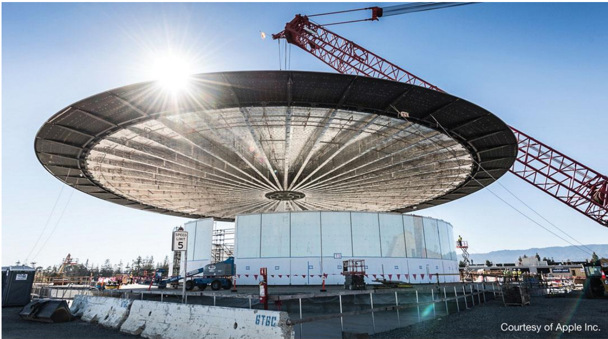
Fig.3: Apple Campus 2, CFK-Dach-Tragwerk, 2017, 80 t, \Phi 52 m.
