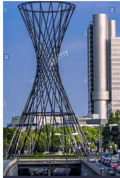
Fig.5: 'Mae West' Munich, 52 m high, CFRP-tubes, Rita Mc.Bride artwork [Alamy-stock photo]
