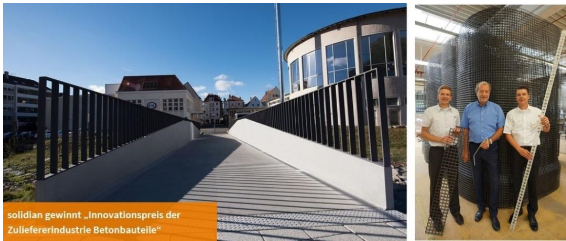
Fig.28: Carbonbeton-Brücke Albstadt-Ebingen, (rechts) vorgeformte Bewehrungsstrukturen [Solidian]. Carbon Concrete Bridge Albstadt-Ebingen, (right) pre-shaped reinforcement structures
