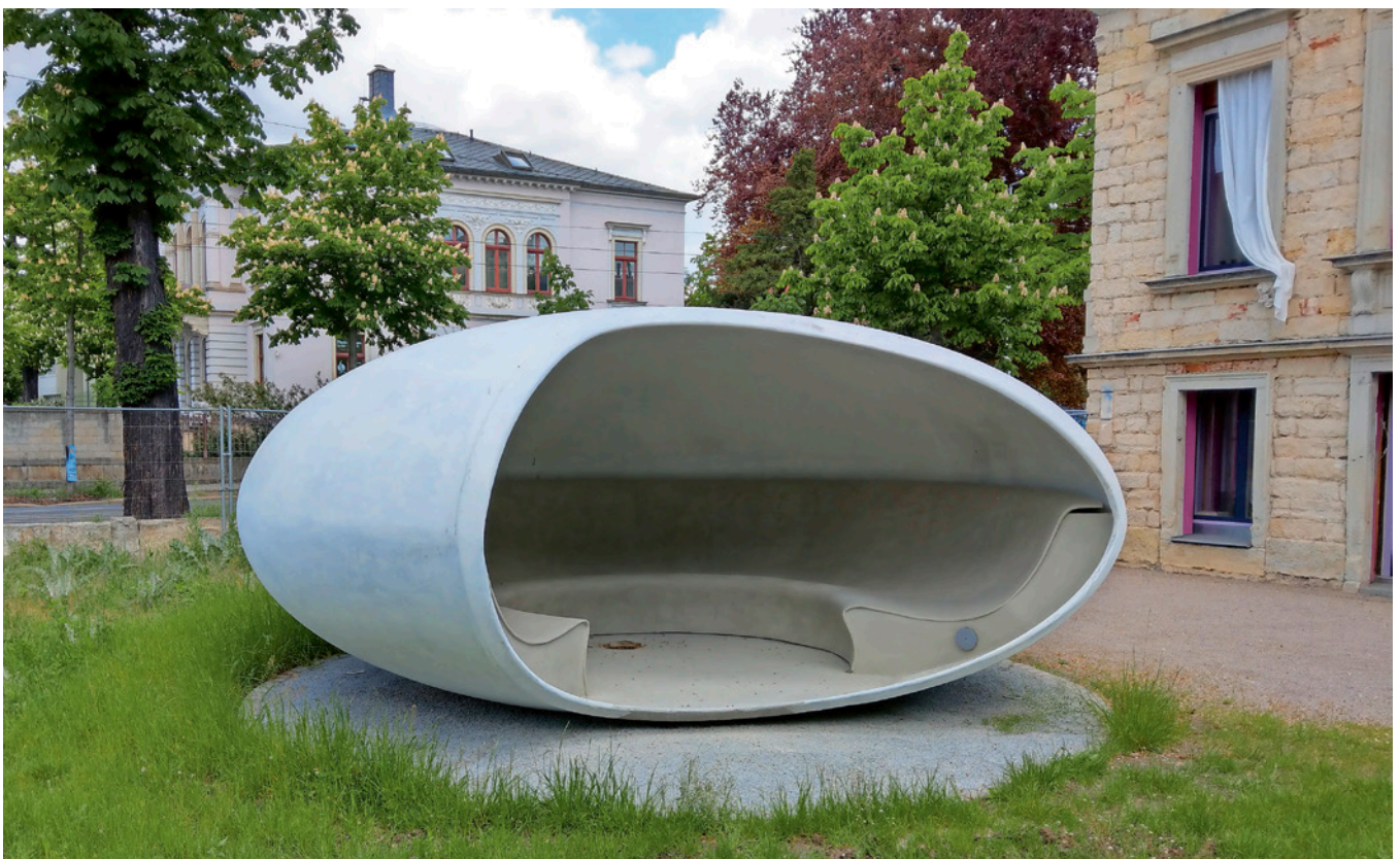
Lightweight pavillion “Smartie” – elegant symbiosis of textile reinforced concrete and efficient design
