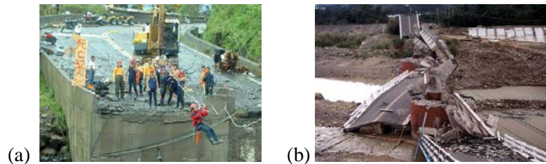
Figure 1. Damage of bridge and disaster relief due to: (a) Typhoon Morakot and (b) Chi-Chi Earthquake.
