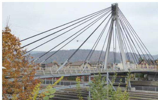
Figure 11. Cable stayed Stork Bridge in Winterthur with CFRP stays.
