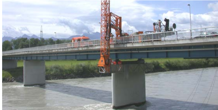
Figure 9. Oberriet Bridge during inspection.
