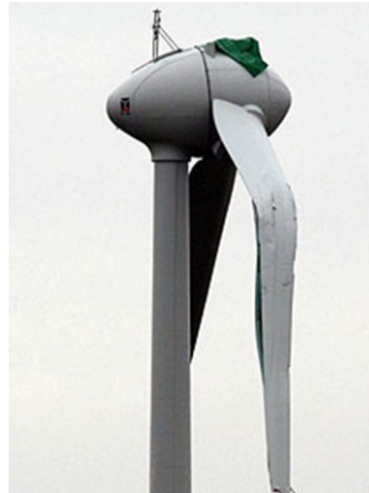
Figure 1 Fatigue failure of a composite rotor blade in Conisholme, Lincolnshire, 2009 [5].
