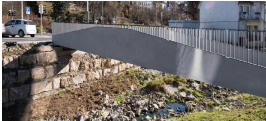
Fig.8-3: Passenger bridge, 2015: Length 15 m, width 3 m, mass 14 t. Erection during 1 night (up) a solidian GRID Q95-CCE-38 fiber grid (mat) [christian.kulas@solidian.com, www.solidian.com ] (down) First, purely CF-reinforced concrete bridge in the world. Albstadt-Ebingen. 2015.
