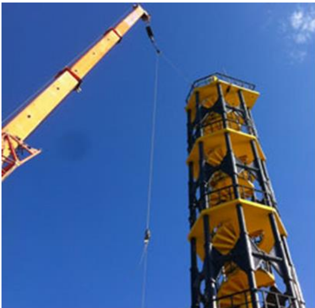
Fig. 8-7: (left) Construction of a 31-m high lighthouse at the Port of Valencia, made from CFRP and GFRP; (right) CFRP tube detail scheme, 2015. José David Jiménez Vicaria MSc Civil Eng., Ignacio Pascual Navarro, Enrique Navarro Lera MSc Mech. Eng., Pablo Sanchez Sierra MSc Mech. Eng. & Eva Martinez Barriguete Chemist (2018) An Innovative New Lighthouse at the Port of Valencia, Structural Engineering International, 28:4, 546-549, DOI: 10.1080/10168664.2018.1464377
