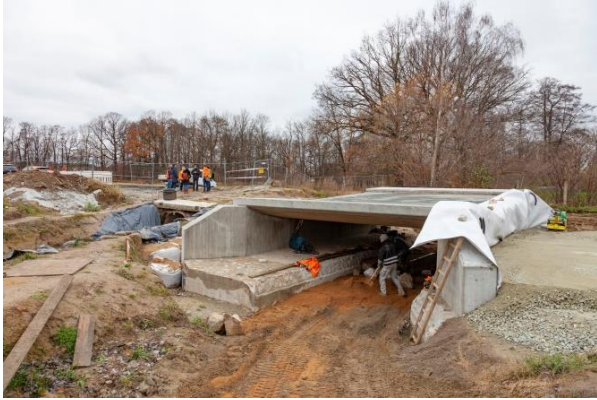
Fig.8-5: Bridge Wurschen, 2022: (left) Superstructure made exclusively of carbon concrete, shell construction. (right) Textile FRP mats in the super-structure) ( Foto: Stefan Gröschel, IMB,TU Dresden)
