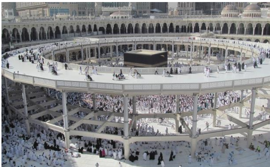
Fig.8-2: Mekkha, CFRP- Pilgrim path construction around the Kaaba. Inner - \Phi 80 m, 400 t CFRP [Premier Composite Technology PCT, Dubai, Vancouver.sun.com]
