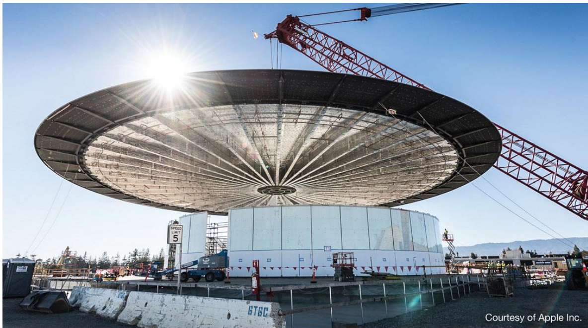
Fig.3: Apple Campus 2, CFK-Dach-Tragwerk, 2017, 80 t, \Phi 52 m.
