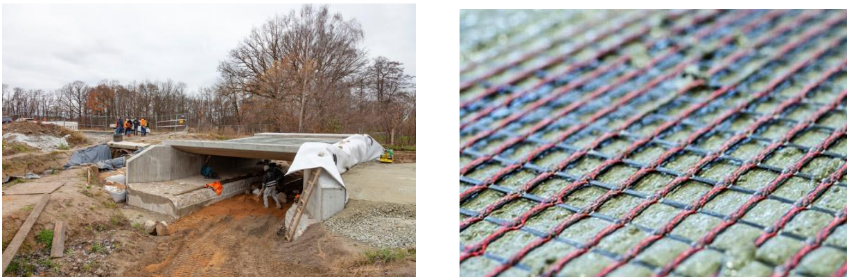
Fig.20-1: Bridge Wurschen, 2022: (left) Superstructure made exclusively of carbon concrete, shell construction. (right) Textile FRP mats in the super-structure) (Foto: Stefan Gröschel, IMB,TU Dresden)
