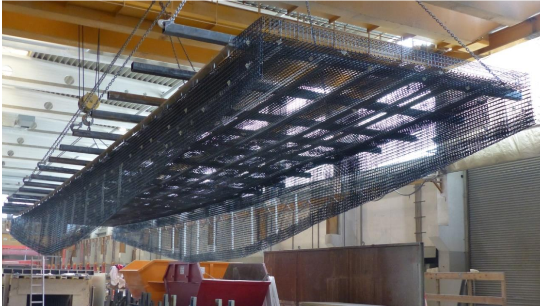
View of the finished reinforcement cage.
