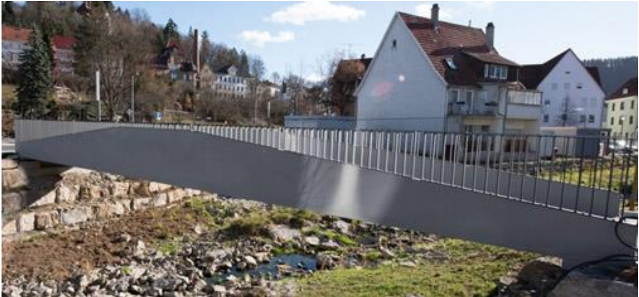
Passenger bridge, Albstadt Ebingen 2018: Length 15 m, width 3 m, mass 14 t. Erection during one night ! [courtesy Solidian]
