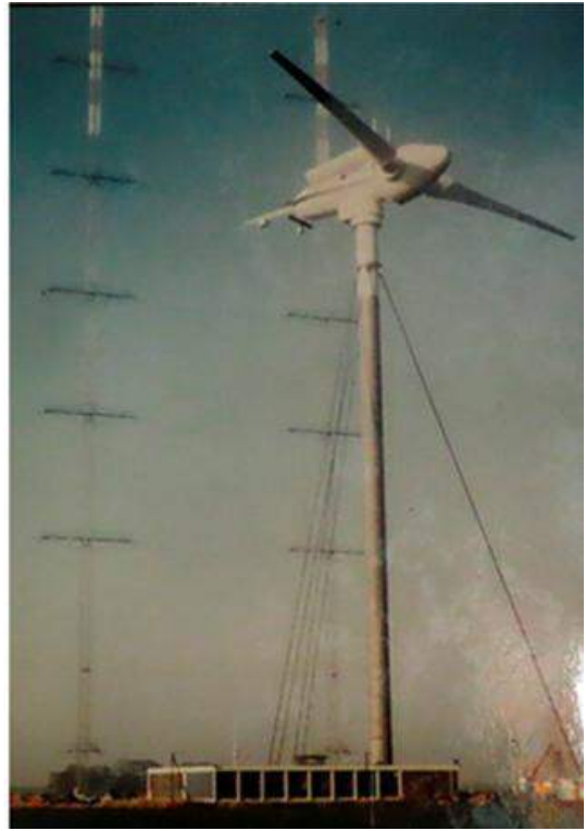
Wind Energy Rotor GROWIAN, 1980, 51 m blade, Profile NACA 44, 3 MW electric power. GFRP shell with wind speed measurement facility.
