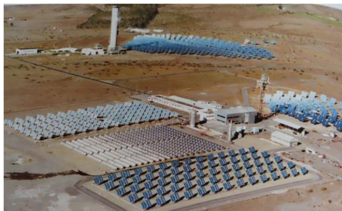
Solar Farm Plant with tower.
