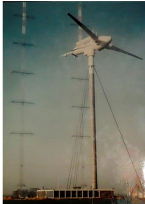
Wind Energy Rotor (GROWIAN, 1980, 51 m blade, GFRP shell ) with wind speed measurement facility
