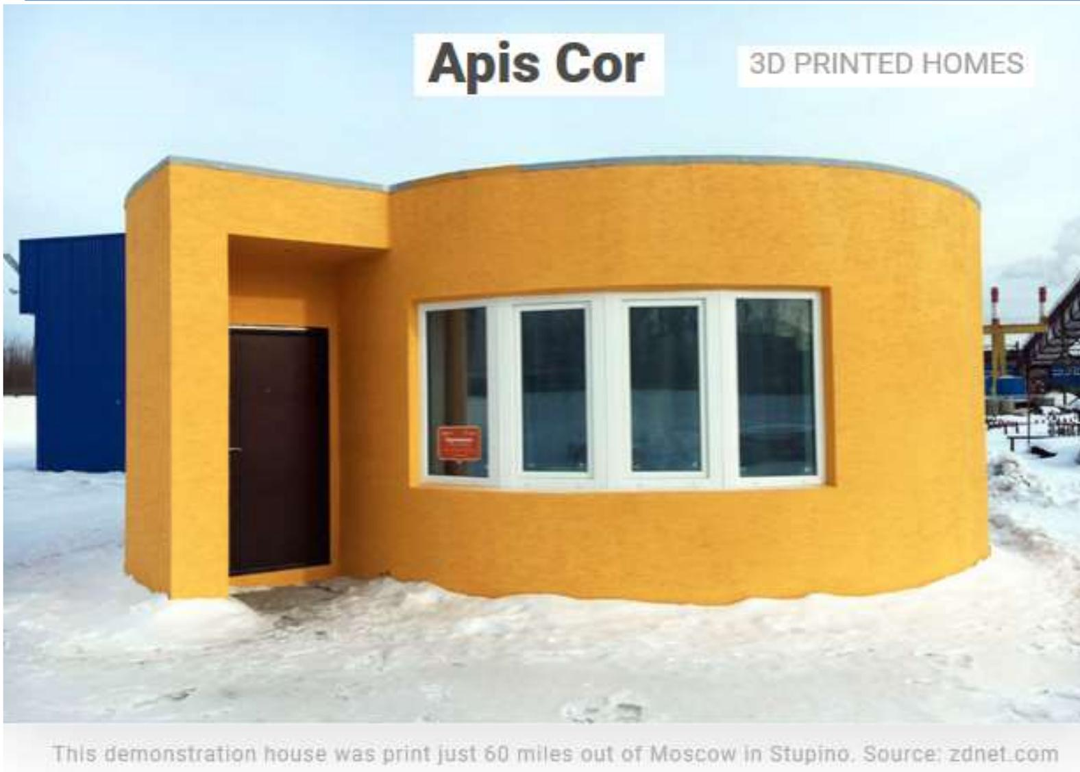
Apis Cor also believes that in the near future homes may be printed using **dual extrusion**, allowing the **insulation** and other main components to be printed alongside the concrete structure. Apis Cor produced a home in a suburb of Moscow in just 24 hours. Source: Maxim Grigoryev / TASS
